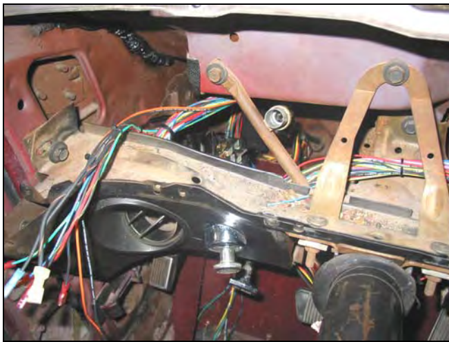
Figure 6-9 Interior Section Routing
