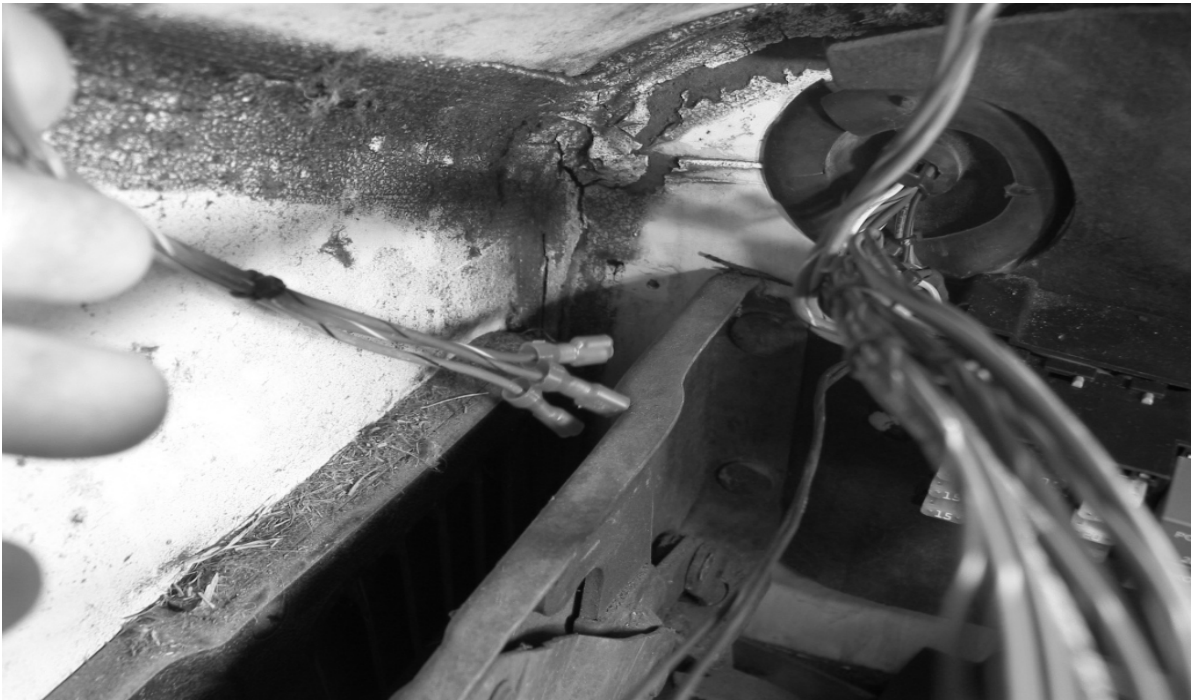
Figure 7-22 Routing the Dimmer Switch Wires
