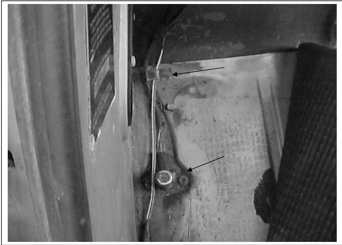
Figure 6.7 Routing of the Cab Section. Down from the fuse block and through the groove in the door jamb. Arrows are pointing at the Dimmer Switch and a mounting bracket.
